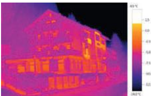
Thermal image with ScaleAssist
